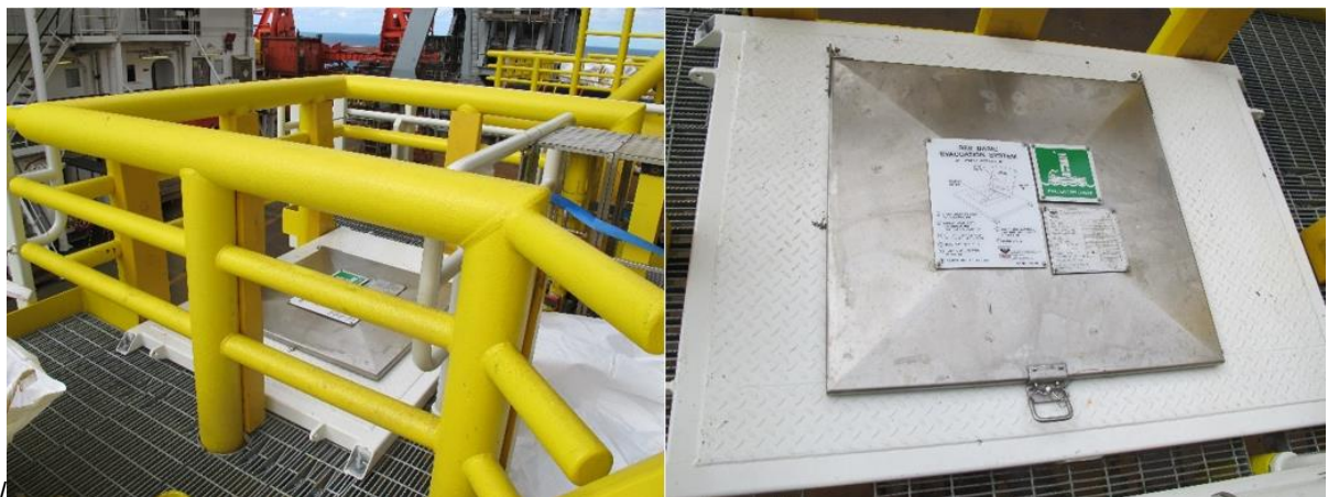
Figure 1. Example of escape chute arrangement
